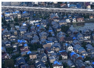
2018 Northern Osaka Earthquake*
